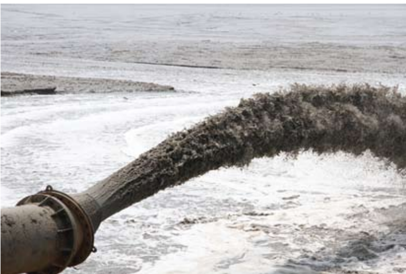
Above: A mud-pumping barge and pipelines. The previous year, this had been one of the best spots to watch knots from. Photo P Battley. Below: A pipeline discharges its mud slurry into a settling pond. Photo P Battley.
