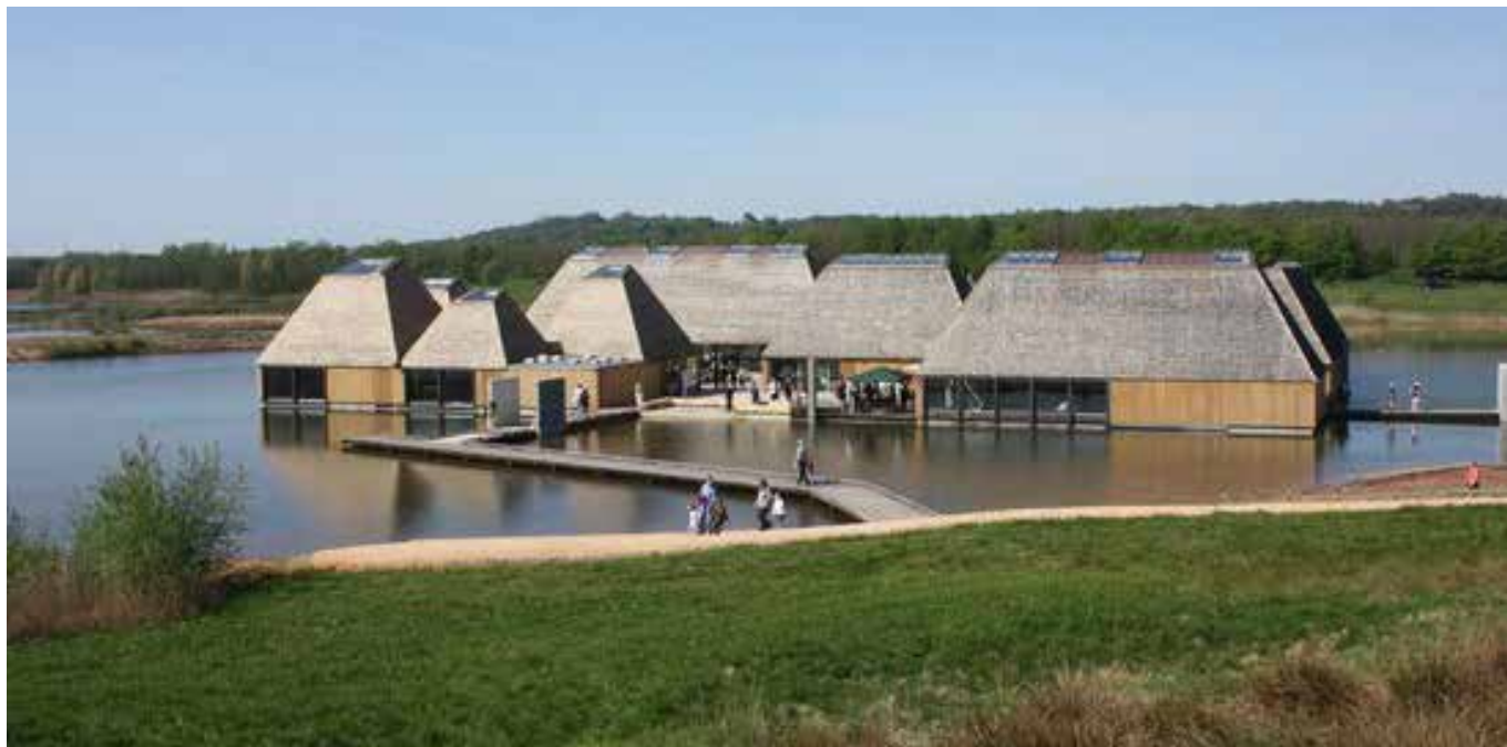
NOT FOR US: This floating visitor centre at Brockholes, in Lancashire, has been suggested by consultants as a possible model for a new Shorebird Centre. But the PMNT Council isn't keen.
